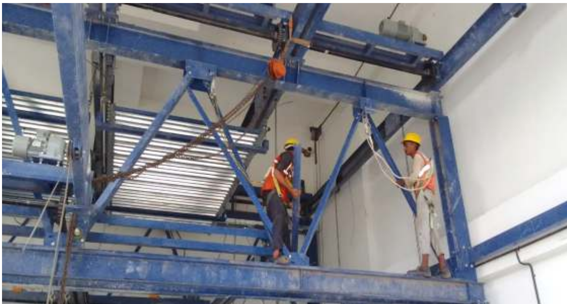
Mechanical parking work in progress.
