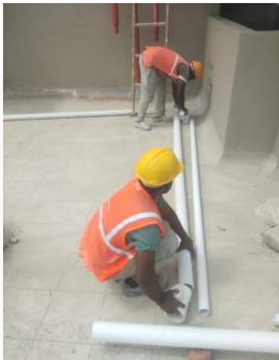
A3 External plumbing work in progress.
