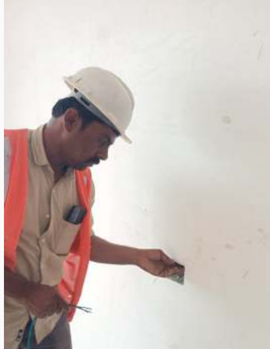
Electrical wiring work in progress on 17 th floor.
