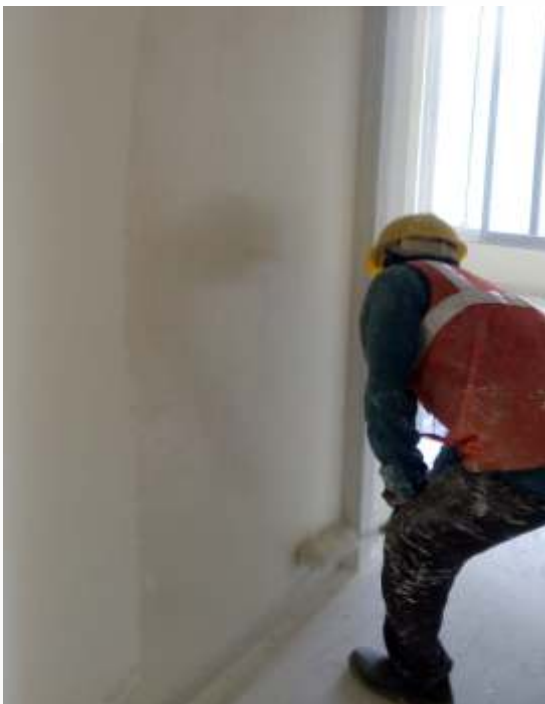
1 st Coat painting work in progress on 13th floor.
