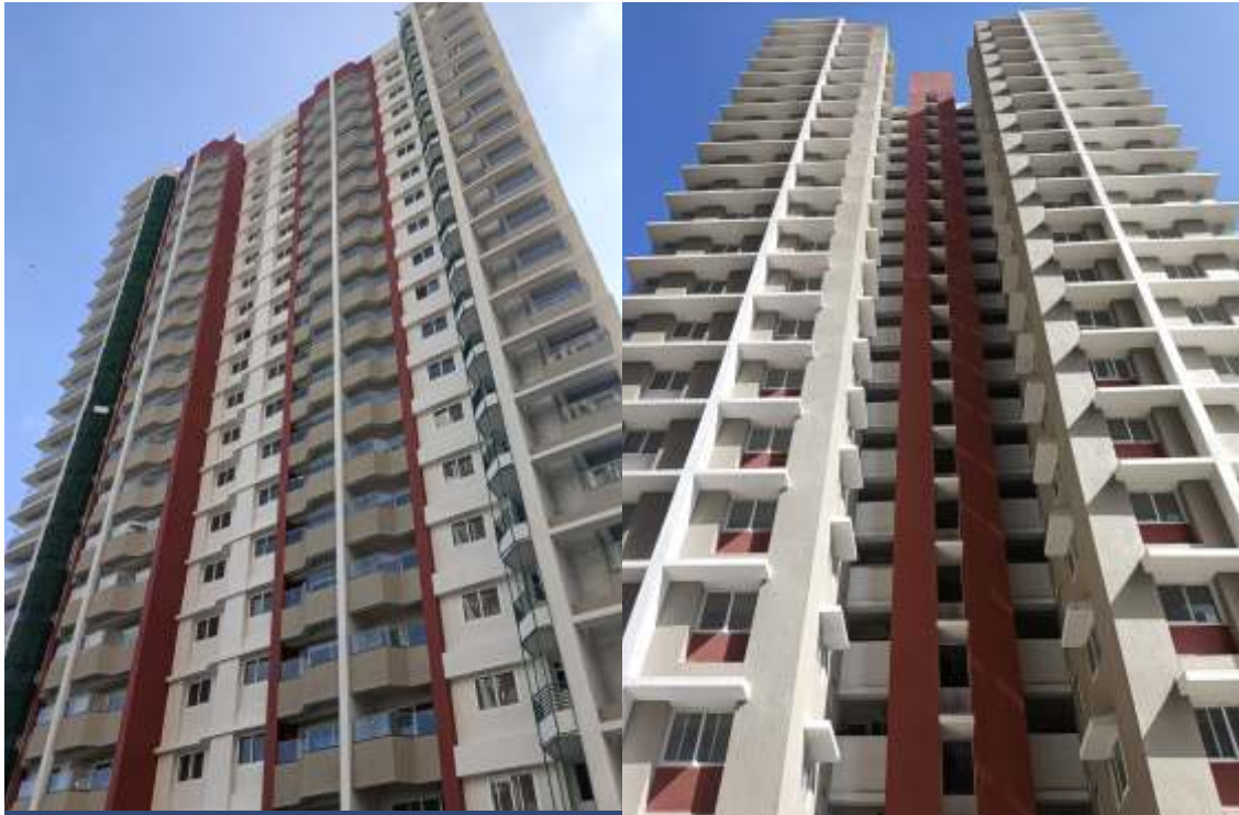
Internal final coat Paint & Snagging in progress.
