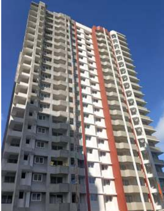
External painting work in progress.
